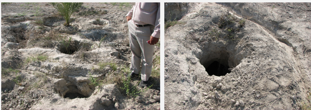
Figures 17 and 18: Existing porous which are similar to holes which more than 1 meter depth.
