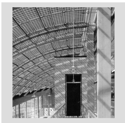
Figure 5. Interior of conservatory with transparent modules at ECN in Petten, the Netherlands, (Prasad and Snow, 2005).
