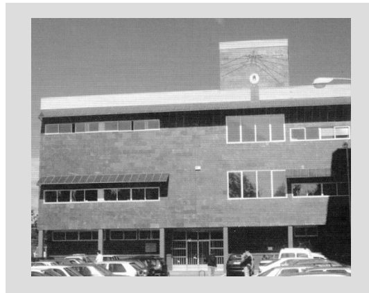
Figure 2. IES building in Madrid, Spain (Prasad and Snow, 2005).
