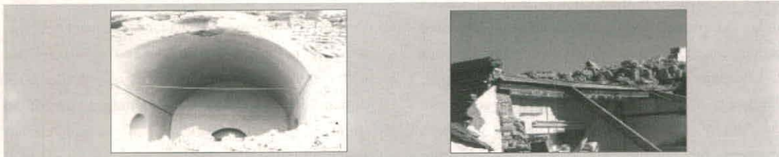
Figure 4- Comparison of stability of steel barrel-vaults and the vaulted-ceilings of mud-brick in Bam Earthquake, and the effect of relative amount of walls
