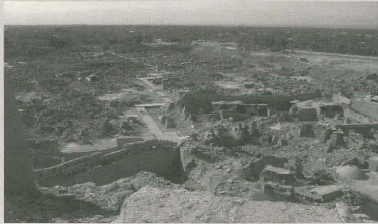
Figure 1 – A view of the destruction from the top of the Citadel towards Bam
