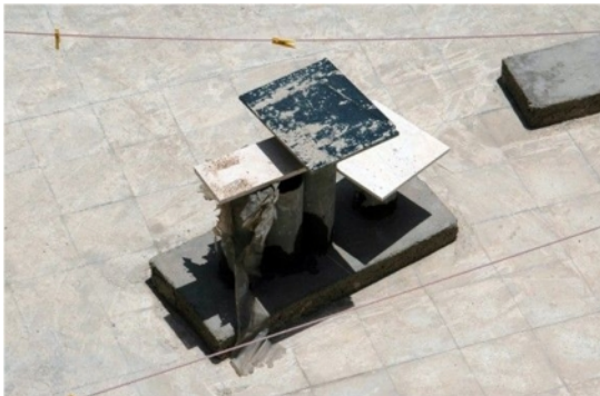
Figures 9 and 10. Flue gas stacks (Shahre, farang.com).
