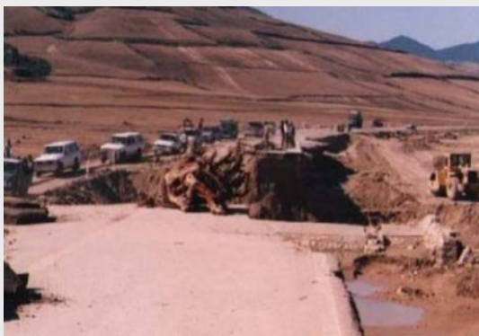
Figure 1- Damage to built-up construction.
